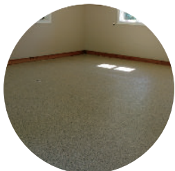
Interior Floor Slabs
